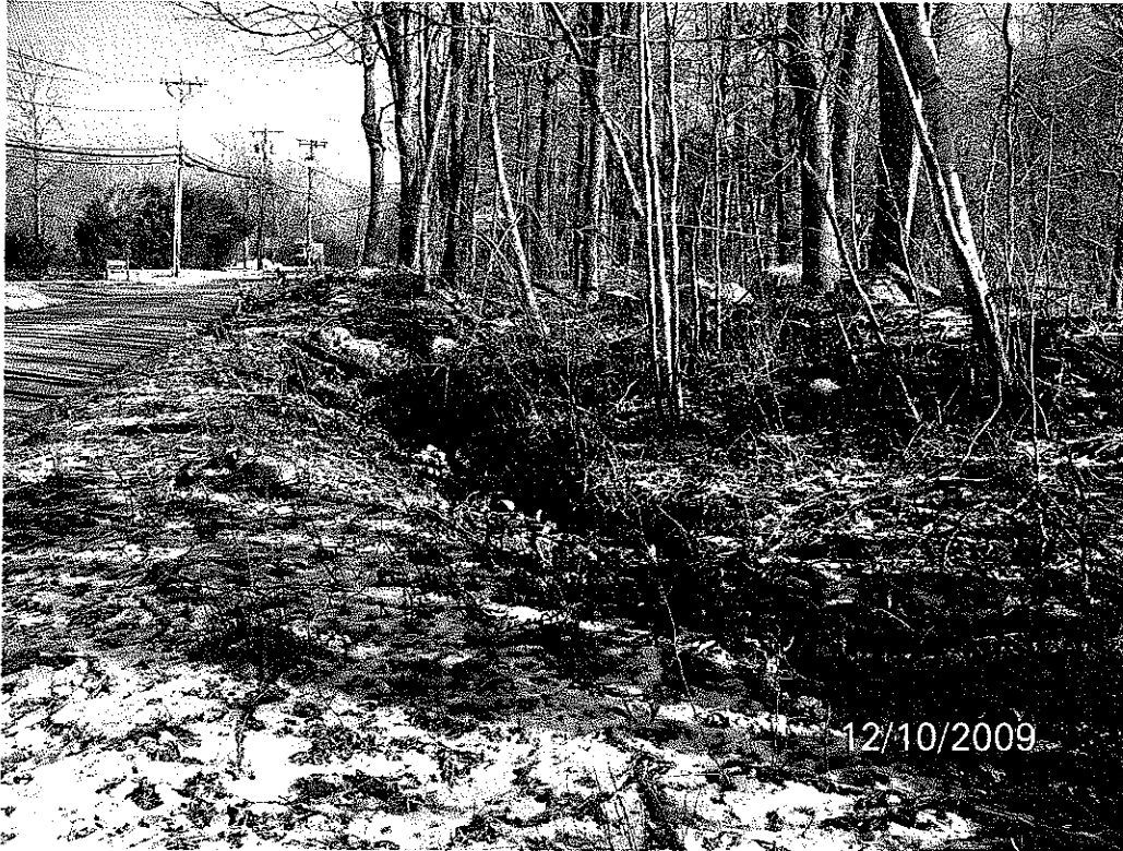
Wetland Site 3: Looking East down Rte 82 Overflow Channel
